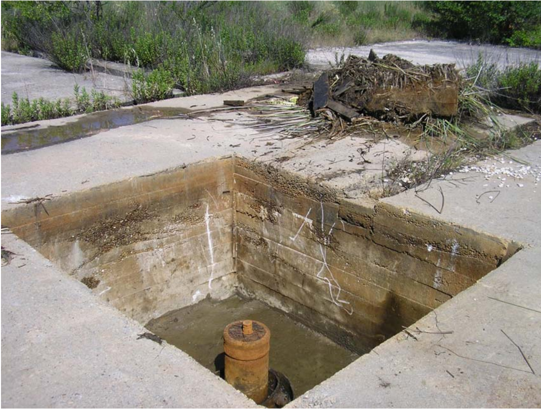
Geo-Madrid well cleared for re-entry and well inspection and testing.
