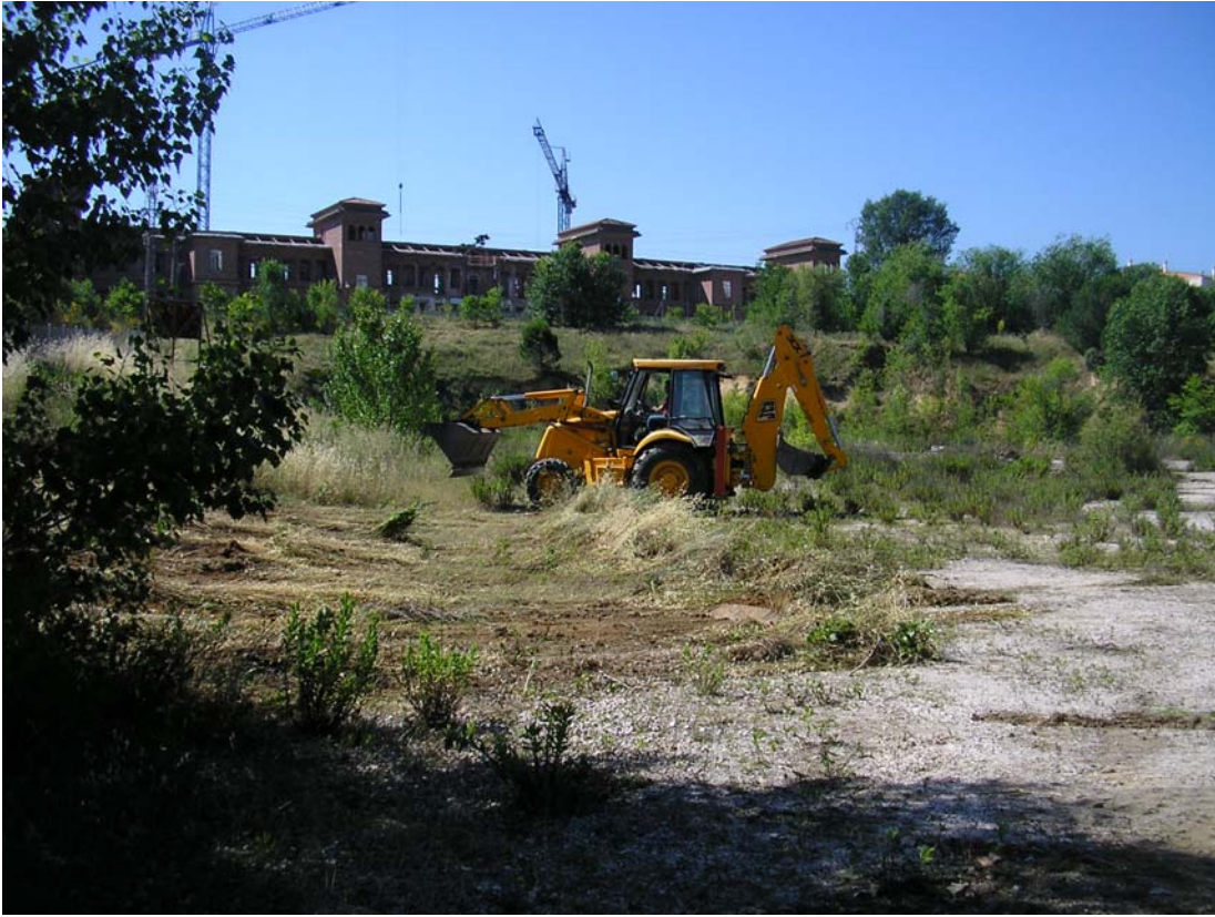
Site Clearance work underway at the Geo-Madrid doublet well location
